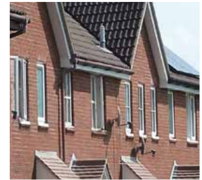
Red brick wall
