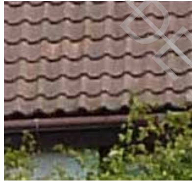
Red / brown concrete pantiles
